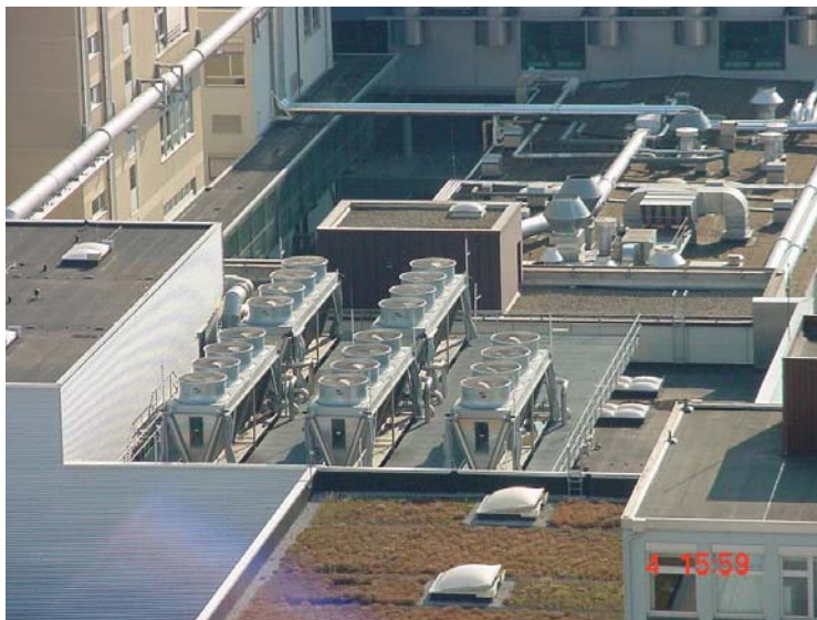
Hybrid coolers in use at an automobile manufacturer for Dynamometer cooling
